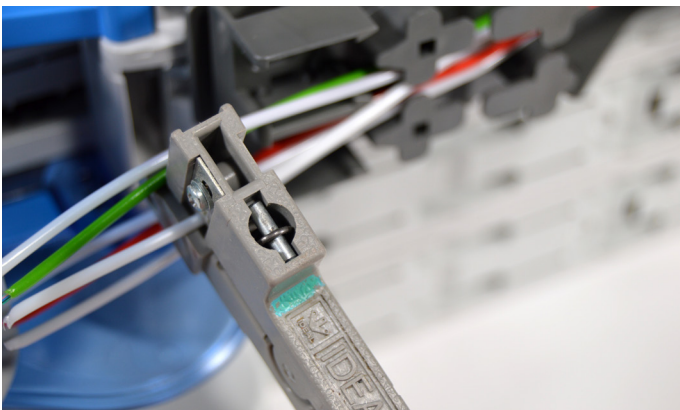
6.1.2. Strip the loose tubes at the marked point and clean the fibers.
