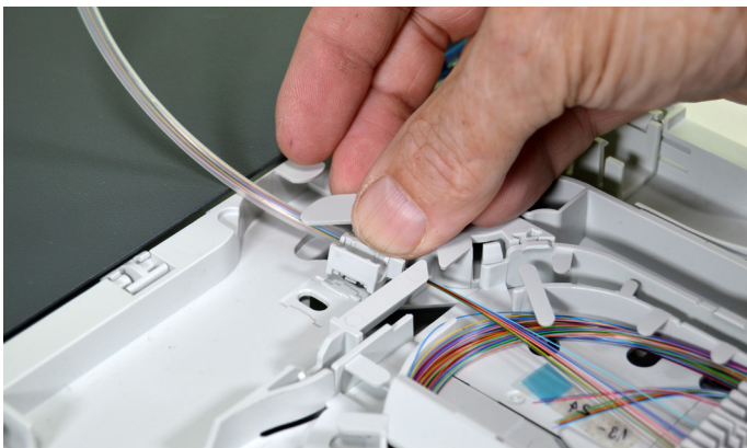
7.2.4. Mount the low tube holder in the tray. A second tube holder can be mounted, if needed.
