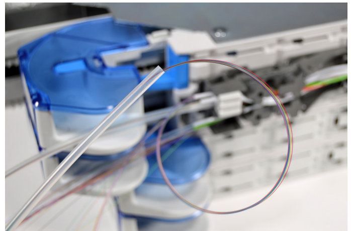
6.1.5. Feed the fibers into the -correct length- transportation tubes.
