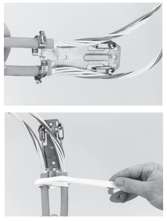
4.1.8 If the cable diameter is more than 8 mm Secure the cables with the hose clamp onto the loop bracket. Wrap a few layers of tape around the hose clamp. If the cable diameter is less than 8 mm secure the cables with tie wraps.
