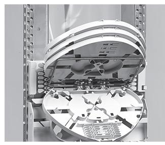
6.6 Identify the tray to be worked on and make it accessible. If the routing block and trays are in vertical position you will have to support the trays above the selected one using the tray wedge which fits in the cavities of the wraparound groove plate. Position the wedge carefully such that the groove is still accessible for the fibers and be careful not to push the wedge against fibers. To remove the wedge, use two hands to pull on both ends (near the groove plate).
