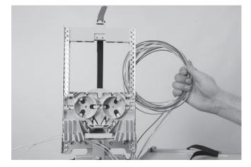
4.1.14 Make some loops with the uncut loose tubes, and put these in the plastic bag (Be careful not to damage the loose tubes!).Two sizes of bags are available. Use the correct size according the volume of the loose tubes.
