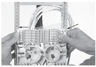
6.2 Secure the wraparound groove plate on the UMS by putting the plate with the long protrusions in the S1 UMS-profile and sliding the plate in the S2 UMS-profile until it snaps. (Do not leave gaps between groove plates).
