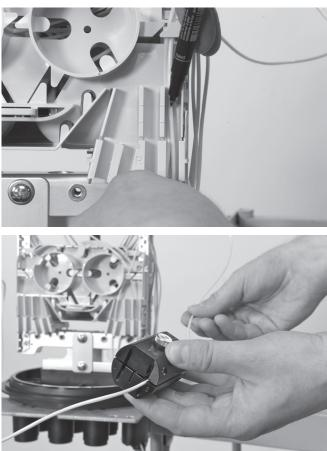
4.1.16 In case of reversed oscillating cable (SZ-cable): separate the loose tube(s). Match the loose tube(s) on the tubeholder and mark both sides between the two marks. Shave between the two marks with the appropriate tooling. Clean the fibers and wind some PTFE tape around the ends of the tubes and fibers ,to protect the transition from tube to fibers.
