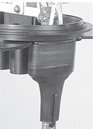
5.1.7 Hold the cable in position. Shrink till the green painting dots become black, and the hotmelt is visible on the end of the sleeve. Postheat the clip on both sides till the adhesive shows a proper flow on the clip between the two cables.
