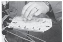
7.1.7 Upon completion of splicing, install the clear protective cover on the tray.
