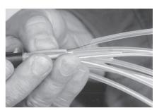
**5.3** Cut the loose tube, at a distance of 35 mm from the cable ring cut and remove and degrease fiber bundle. Select a transportation tube which fits over the loose tube. Slip transportation tube over fibers and the loose tube.
