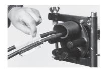
**6.4** Match the blue line of the aluminium cable protection foil with the marks on the cables. Wrap aluminium cable protection foil around cable.
