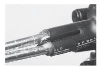
**6.7** Shrink down the end of the sleeve on the cable side. Heat until the sleeve shrinks down on the cables and take care that the green thermo-indicating paint is converted to black. Postheat the clip on both sides till the adhesive shows a proper flow on the clip between the two cables.
