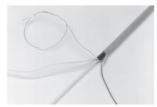
**5.2** Order the FOSC-A-SHIELD-CON-KIT if a shield continuity is required. Cut cable sheath axially for 25 mm from cable ring cut. Crimp shield clip on cable sheath with pair of pliers.
