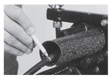
**11.8** Place cable seal over the drop outlet of FOSC base. When cable seal butts against the base, mark the sleeve length on cable sheath.
