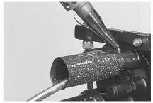
11.10 Slide the cable seal over the port. Shrink the cable sleeve on the base side with the recommended hot air gun device. Use the reflector to ensure heat distribution around the outlet. Shrink sleeve until the green thermoindicating paint is converted to black. Note: setting thermogun: FACC-HEAT-GUN-220V in position 10. Minimum hot air temperature should be 350°C.
