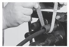
**11.7** Abrade port and cable sheath circumferentially on the cleaned area with the abrasive strip. Remove any abraded material with a clean cloth.
