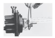
**10.3** Remove gently the sealing ring. Keep the sealing ring and seal area of the closure free of dirt (if needed rinse with clear water).
