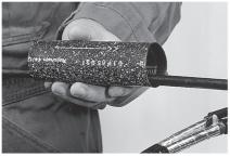
11.2 Remove any dirt, mud or other contaminants from the cable sheath for approximately 2 meters with a clean cloth. Take the cable seal sleeve from the kit FOSC-A-CSEAL-1-NT and slide it over the cable. The non-coated edge of the sleeve and the arrows should be pointed to the base of the closure.
