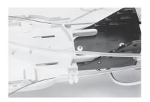
7.1.2 Carefully cut the transportation tubes at the mark and secure to splice tray with two tie wraps. The transportation tube may not be in contact with fibers stored in the organizer.
