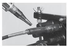
11.11 Shrink down the end of the sleeve on the cable side. Heat till the sleeve shrinks down onto the cable and the green thermo-indicating paint is converted to black. A ring of red adhesive should be visible at the cable on the end of the sleeve.
