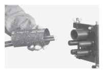
**4.3** Remove any dirt, mud or other contaminants from the cable sheath for approximately 2 meters with a clean cloth. Take the oval cable seal and slide it over the cables. The non-coated edge of the sleeve and the arrows should be pointed to the base of the closure.
