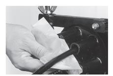
**11.6** Thoroughly clean port and cable sheath with the cleaning tissue over a distance of 100 mm from the edge of the port.
