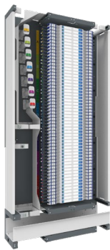
Figure 4: Single frame, recommended patch cord length for all cross-connects is 5 meters (17 ft.).
